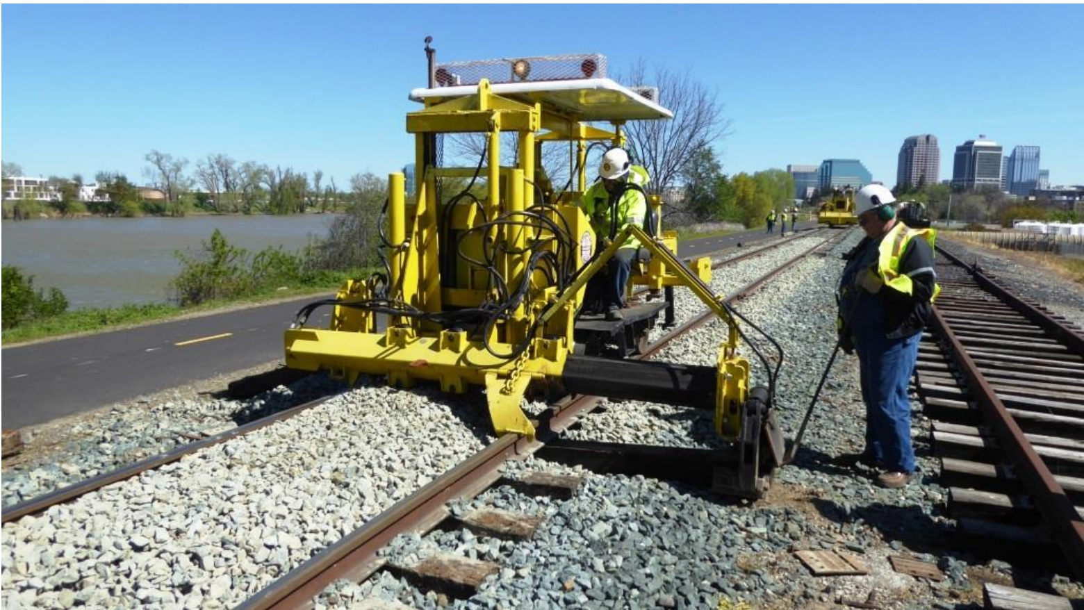
Oops! We missed one. Luckily Joe had the 125 and an extra tie to quickly insert
