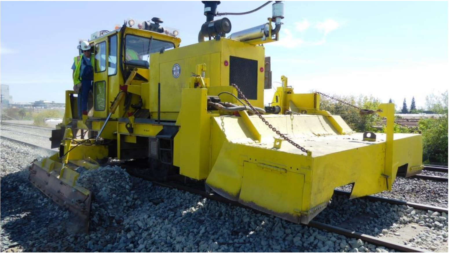
With the regulator's wing deployed, rock is pulled up along the side of the track to form a nice even slope
