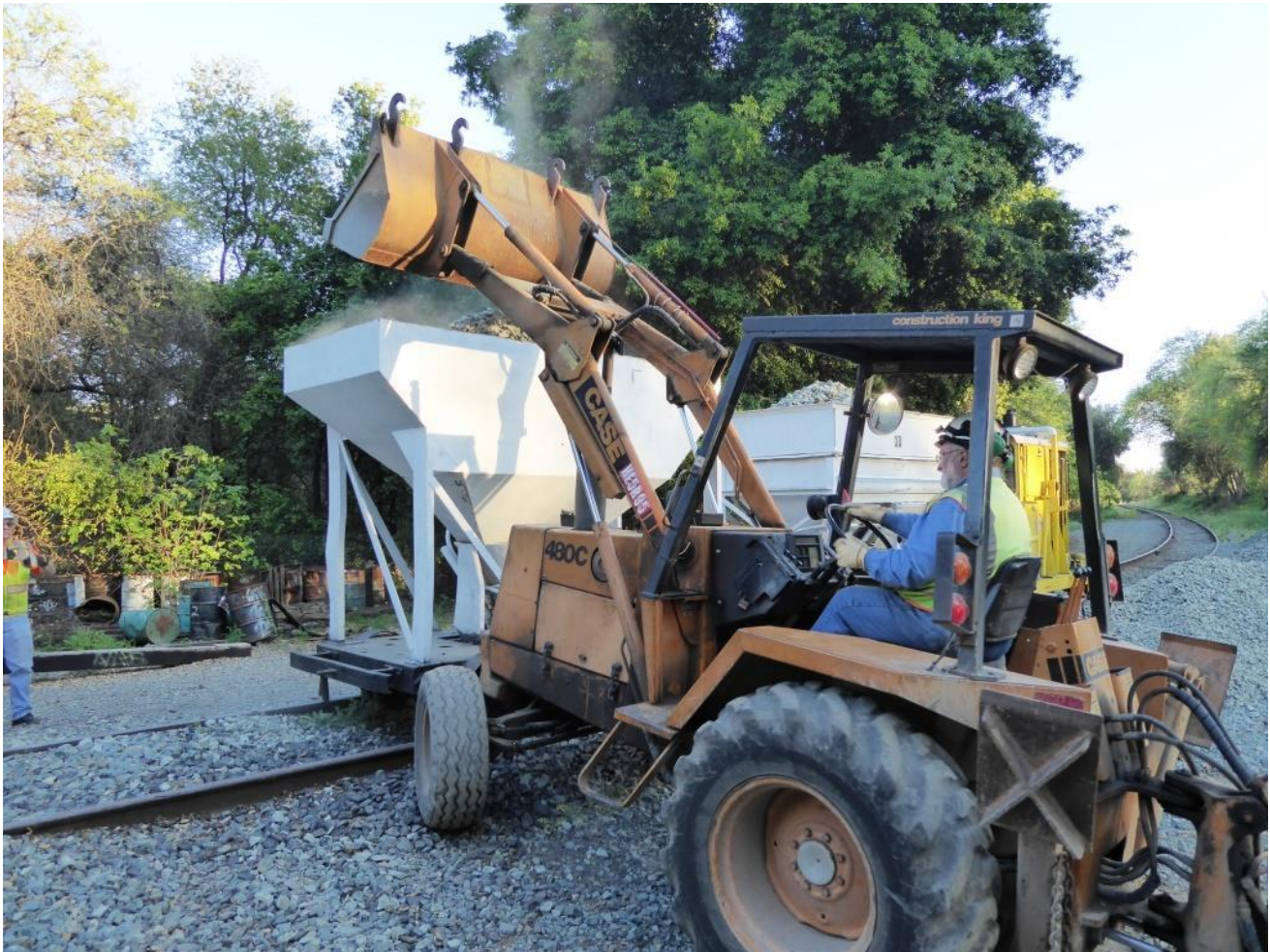
Déjà vu all over again as Frank loads more rock on Thursday
