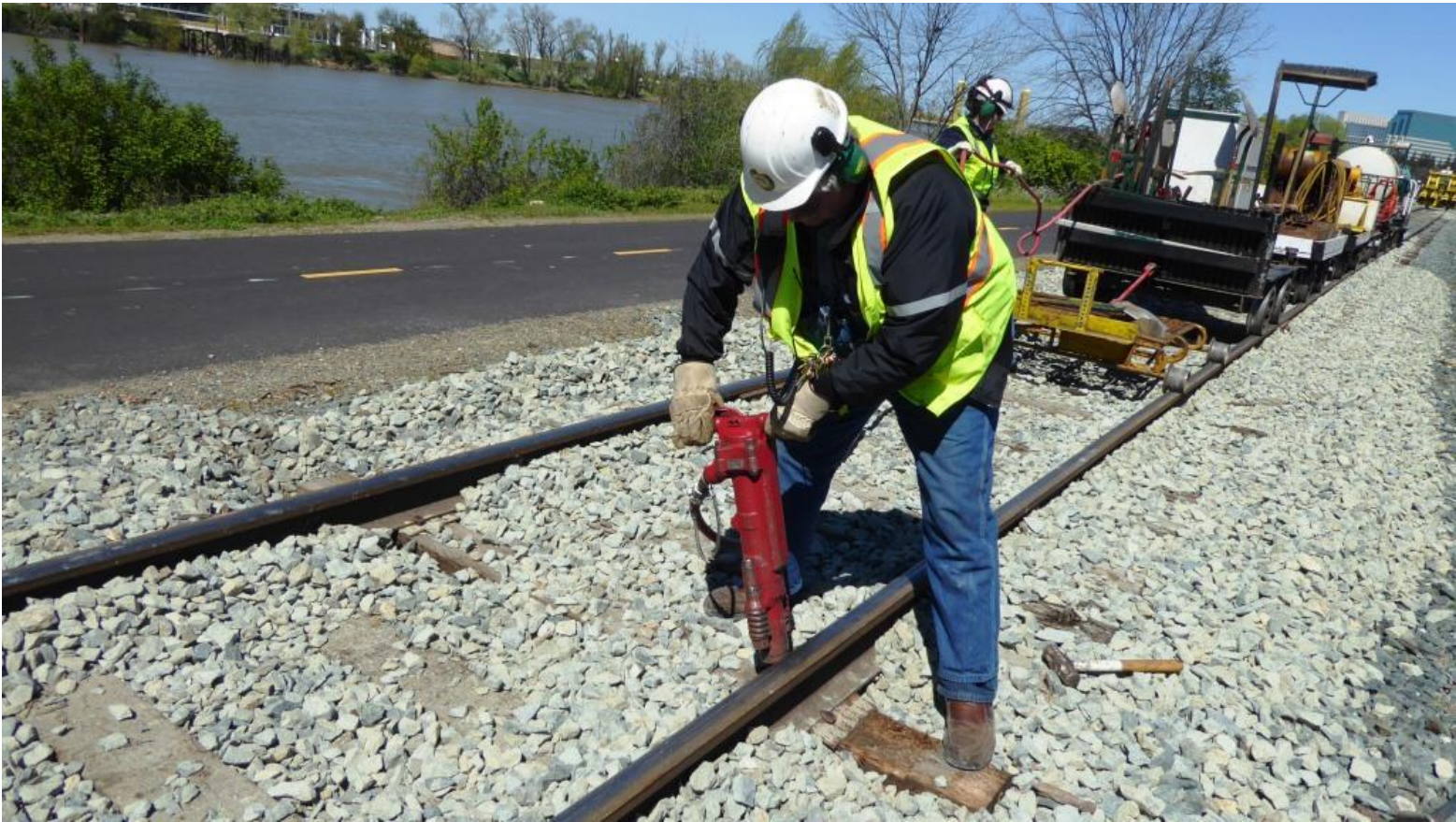
Chris drives spikes with the pneumatic spiker
