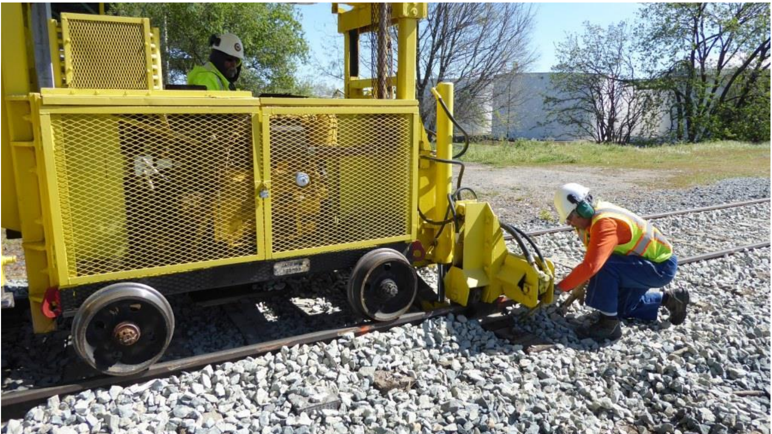
Joe uses the 125's rail-clamps to lift the rail slightly so the Ed can insert a tie-plate
