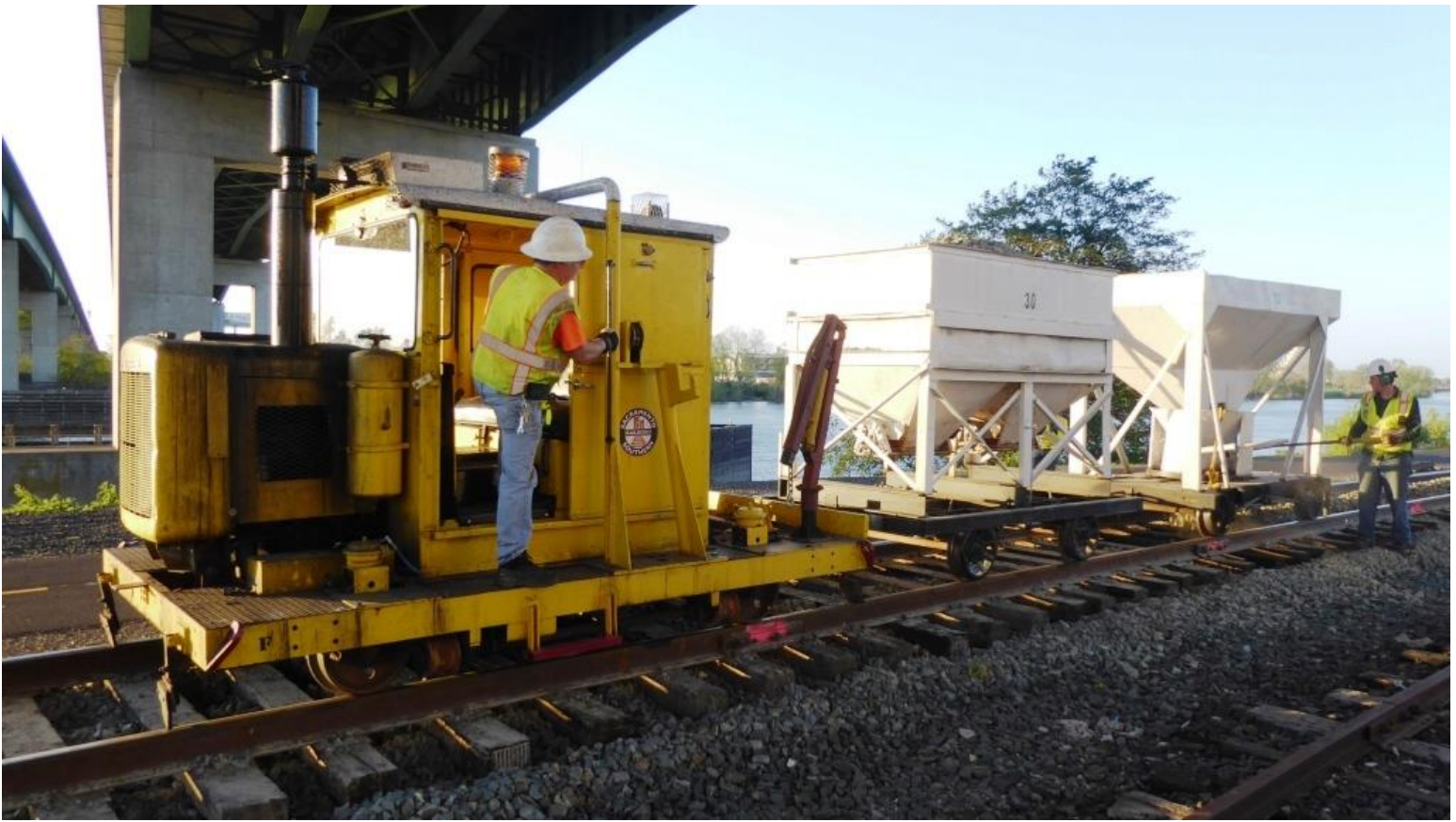
Mike H. pilots the Kalamazoo as Weston drops rock from the hopper
