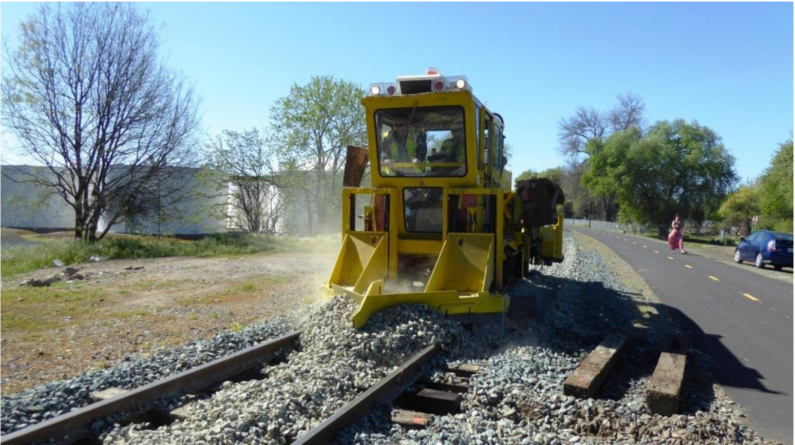
The great monster of the railroad: the ballast regulator plows newly laid ballast rock
