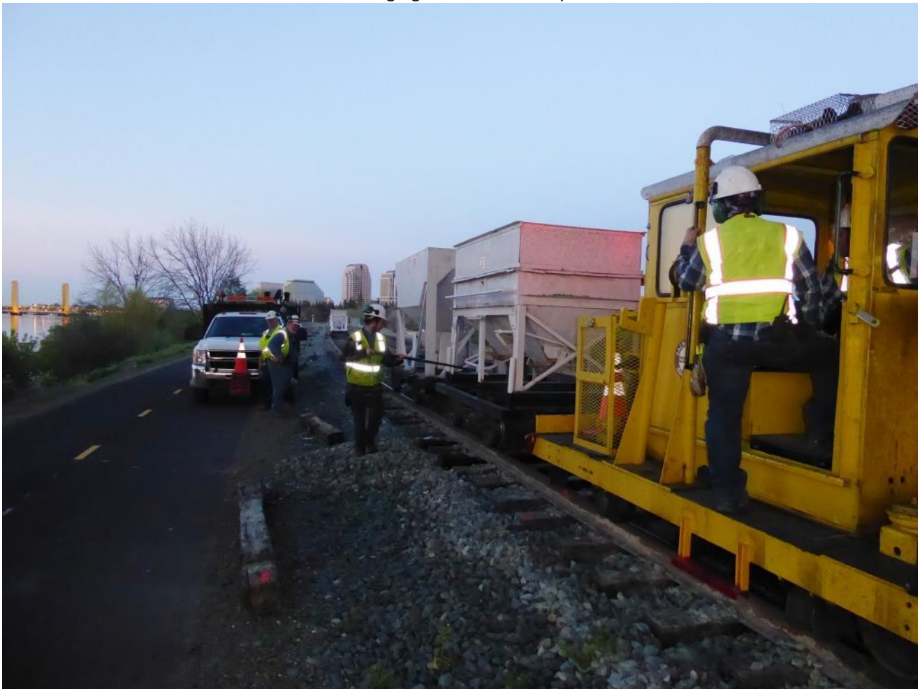
Matt drops rock between the rails just under the Pioneer Bridge
