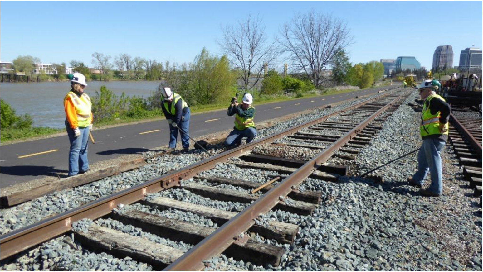
Chris and Mike W. nip a tie up against the base of the rail as Weston sets a spike
