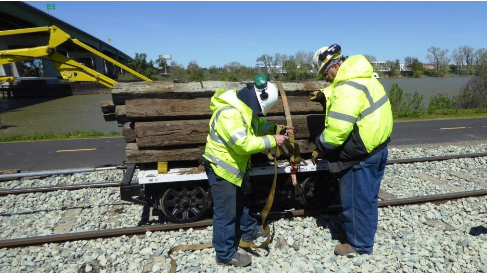
Joe and Mike F. strap down a bundle of dead ties
