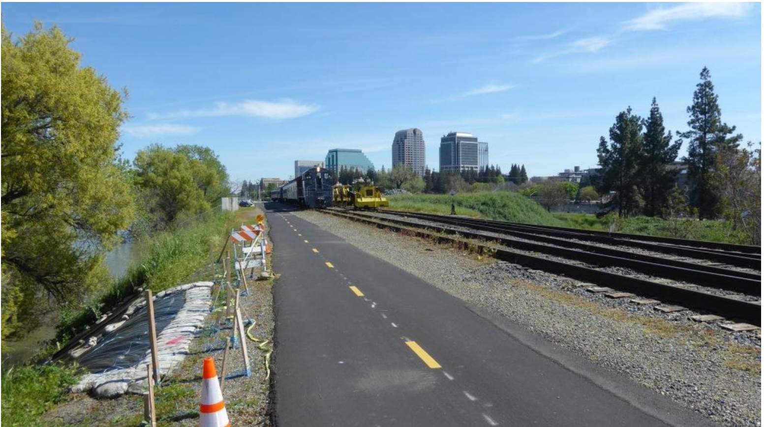
It's train time! The first train of the 2017 operating season passes through the MOW Team's work site
