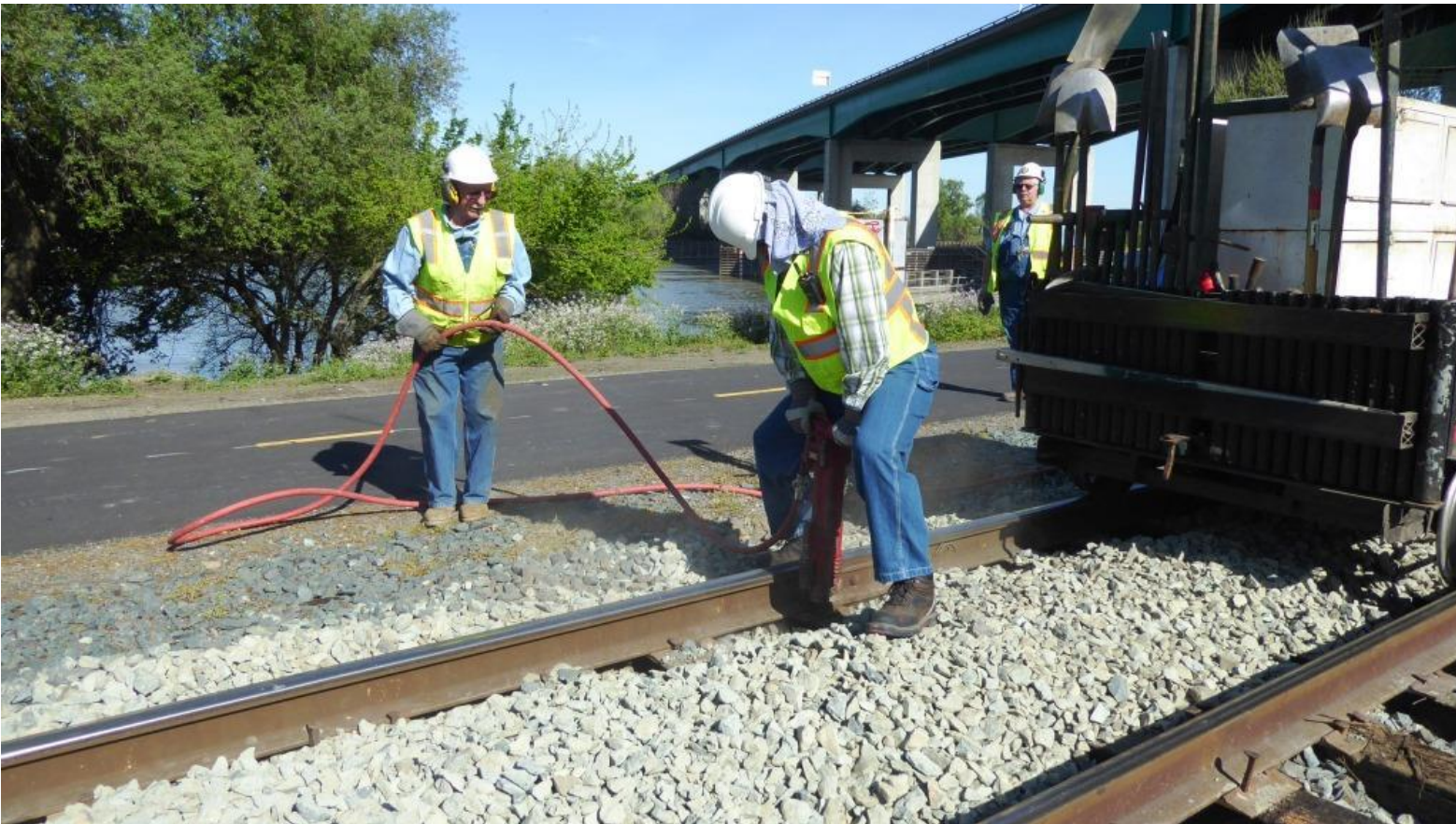
Jose then uses the pneumatic spike driver to drive them home
