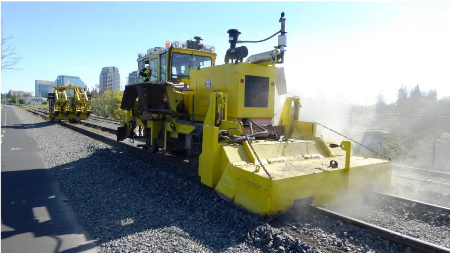
Ed and Chris broom the track with the ballast regulator
