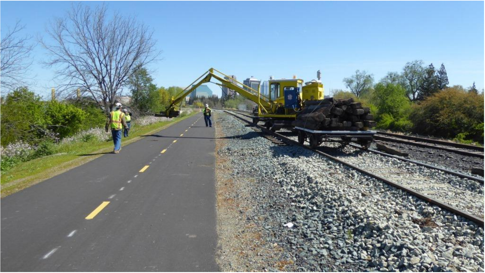
Mike F., Heather, and Clem protect the bike path as the tie-crane's boom swings out over it
