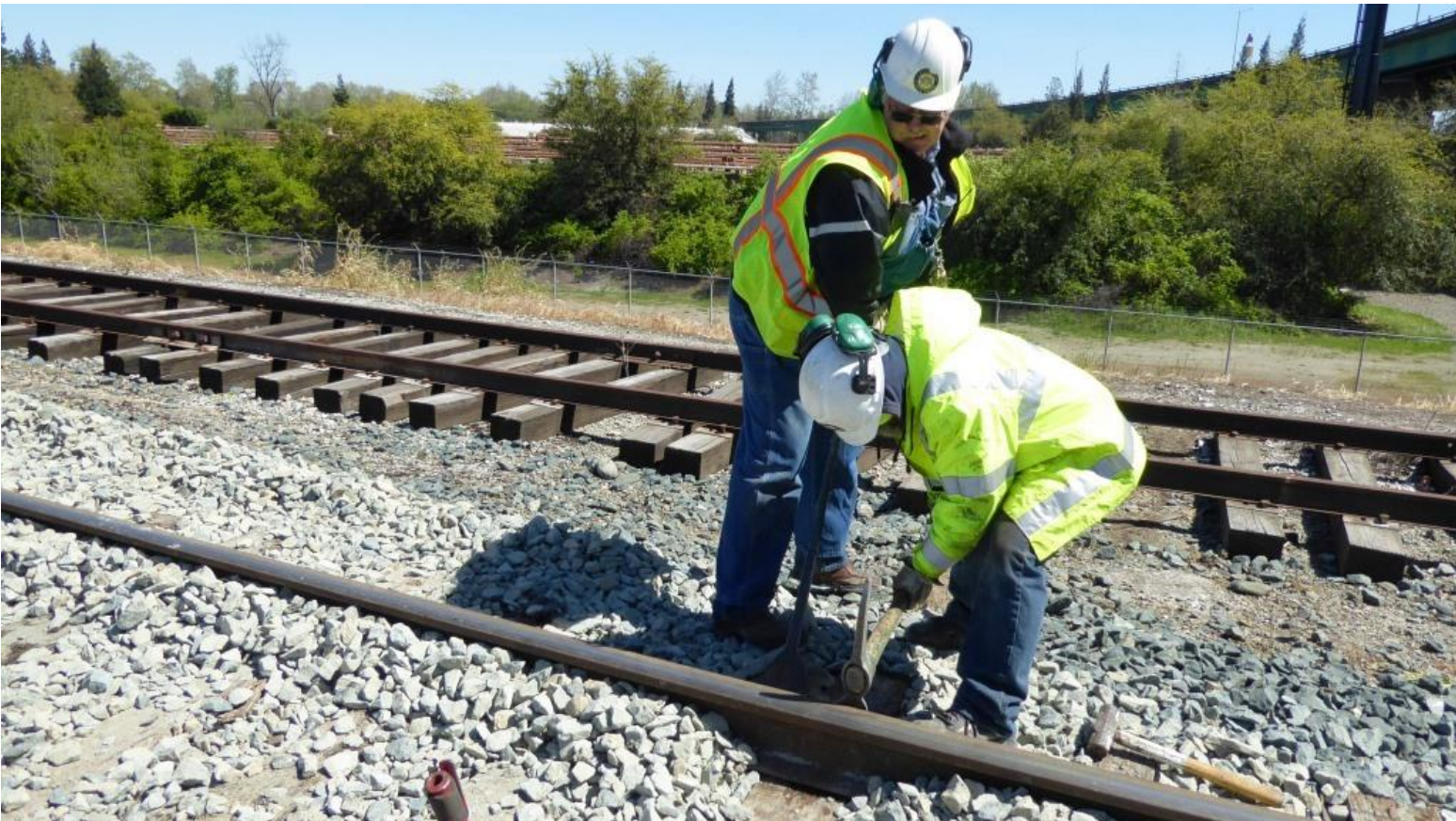
Chris and Joe struggle to straighten a bent spike
