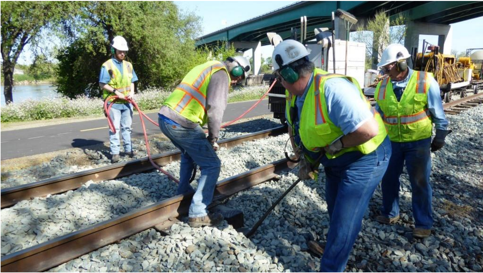
The action picks up as Steve drives spikes while Chris nips the tie
