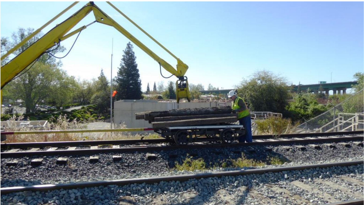
As the tie-crane places ties on the flatcar, Clem adjust them and makes sure they won't fall off
