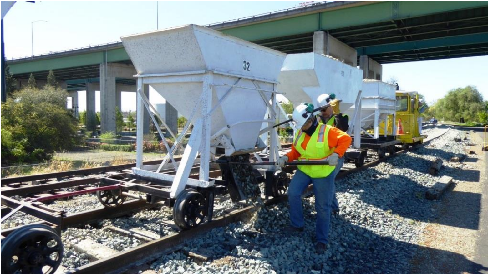
Still lots of holes in the rock to fill in. Bev and Mike W. lay rock along the sides of the track
