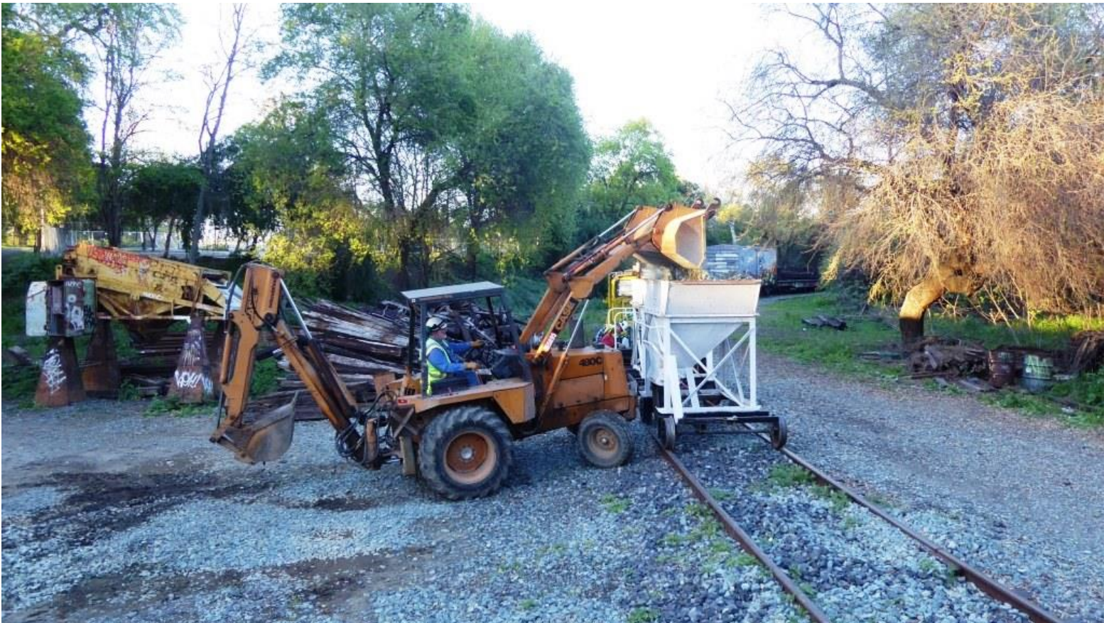
Frank on the back-hoe loads rock into ballast hoppers
